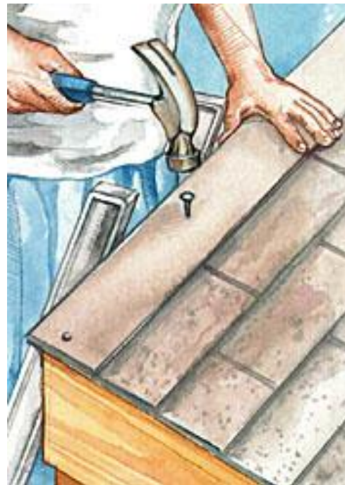
Install shingle courses up to the rear edge, then finish the edge with cut shingles or a solid starter strip.
